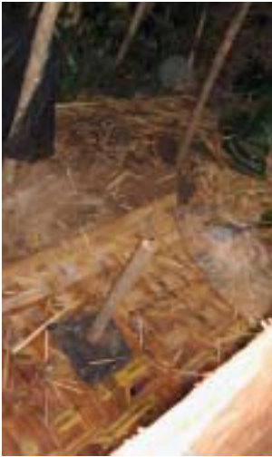
LEFT A direct pit latrine constructed immediately after triggering of CLTS in Uletana Bakole village near Arbaminch in Ethiopia. Notice the use of bamboo, mats and plastic which are locally available materials in construction. Often latrines are gradually improved.
