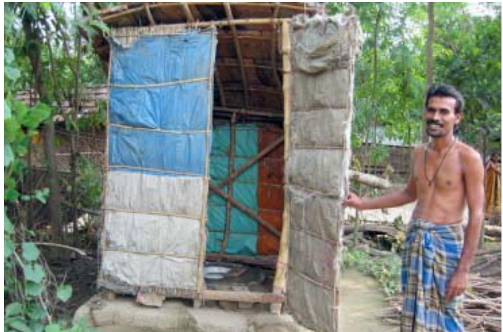
ABOVE Use of bamboo and plastics in making the super structure while the sub structure is strong and perfect. Vidyasagar colony, Kalyani, West Bengal India.
