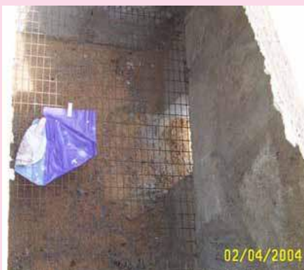
Fire grill inside incinerator
