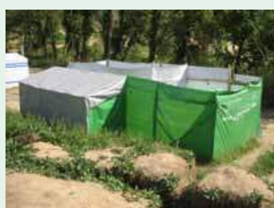
Screened latrine and bathing unit with internal menstrual slab and raised sides for additional privacy
