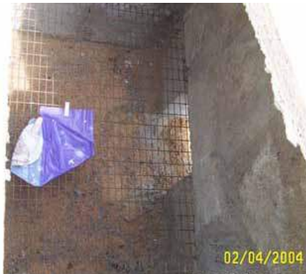
Fire grill inside incinerator
