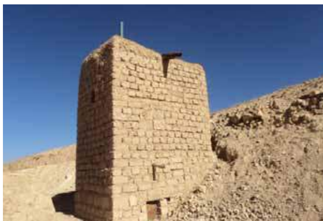
Raised urine diversion pit latrine with urine pipe exit exposed to the atmosphere, Afghanistan (Photo: ACF, Afghanistan)
