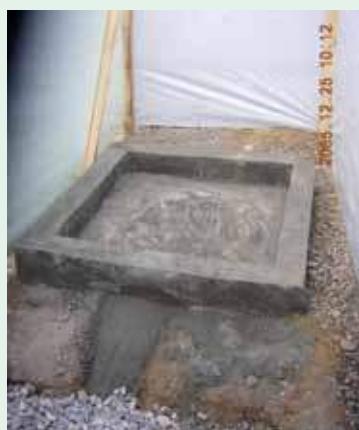
Sanitary pad washing slab inside screened unit
