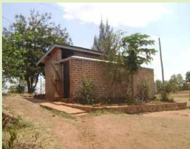
Example of a well-designed latrine with privacy wall
